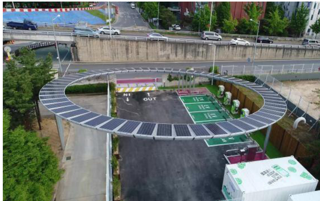
Figure 6: The SMG has installed an EV charging station using waste batteries and solar panels. Credit: Seoul Energy corporation.
